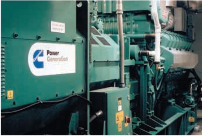
The Cummins Power Generation lean-burn generator set produces up to 1.75 MW of electricity and 4,000 pounds of steam per hour in a CHP application.
